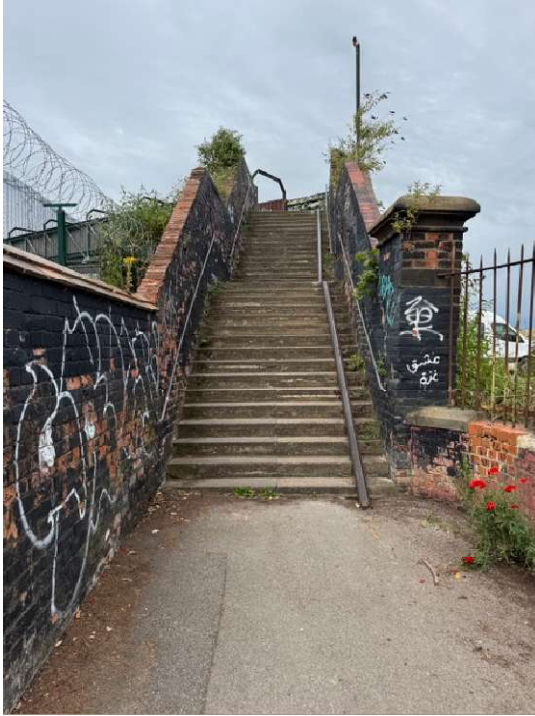
Existing access from Cinder Lane
